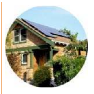
Residential Solar Systems
